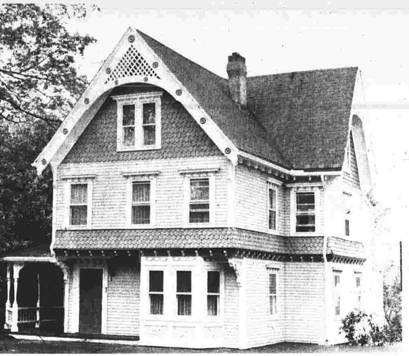
Three-family Victorian house has beige aluminum siding, rust-colored shingles on front and sides, white trim and a blue door. Located next door, not pictured, is the Weiss Gallery.
